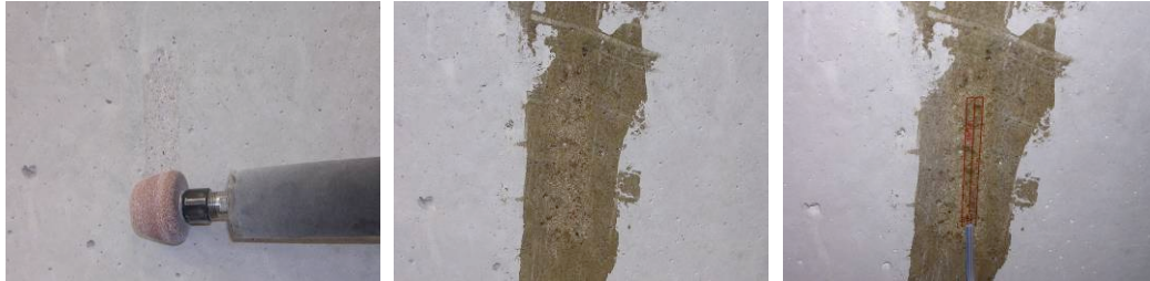
Figure 3-23. Installation of a concrete surface gauge for measuring concrete strains.
